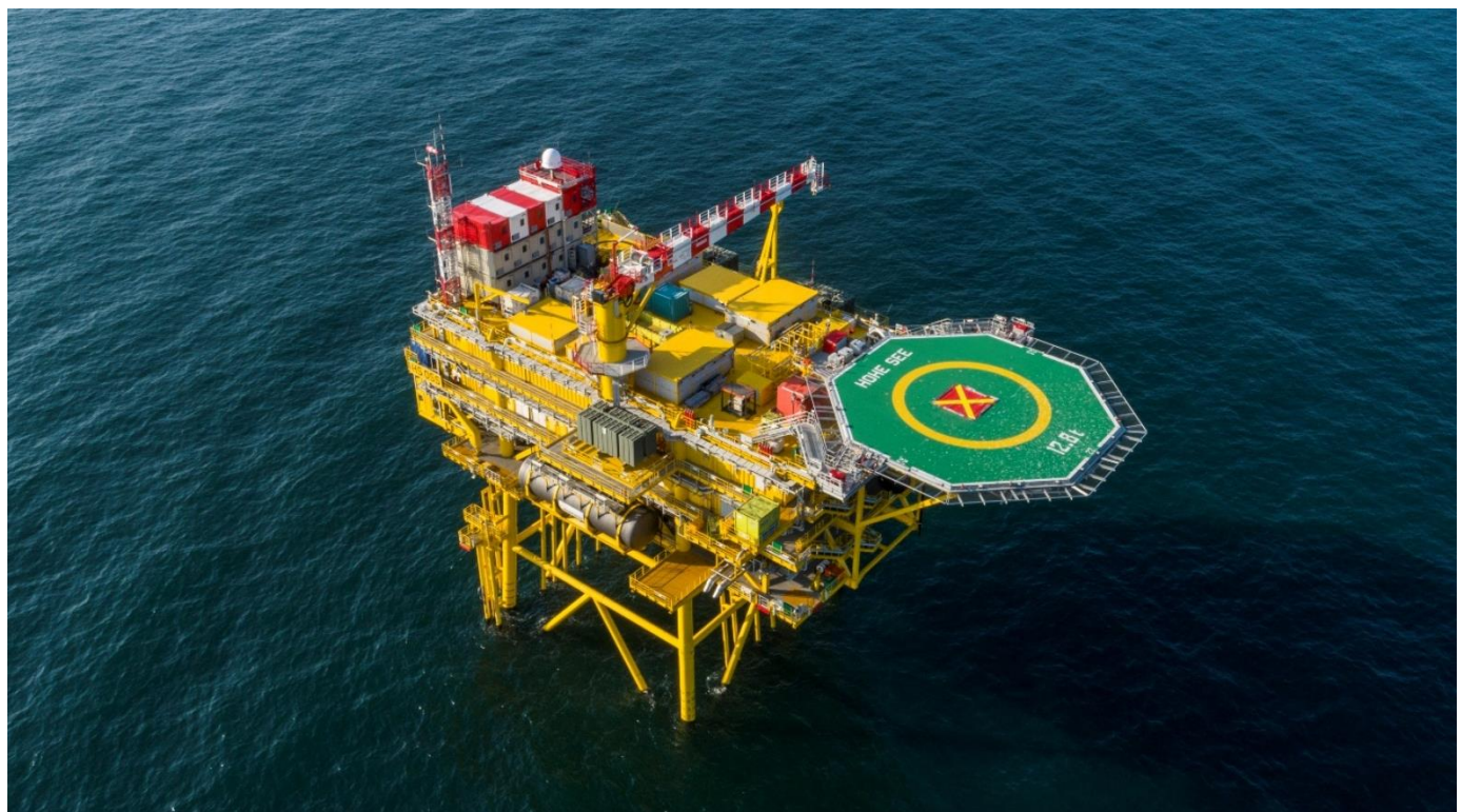
Figure 3.5: OSP at the EnBW Hohe See Offshore Wind Farm in the German North Sea.
